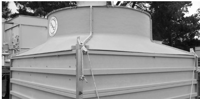
Figure 14: Access Door Anchor Points.
