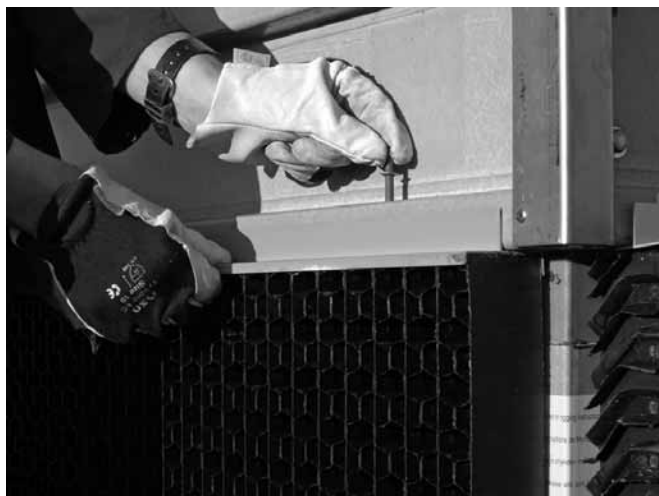
Figure 12: Remove Combined Inlet Shields
